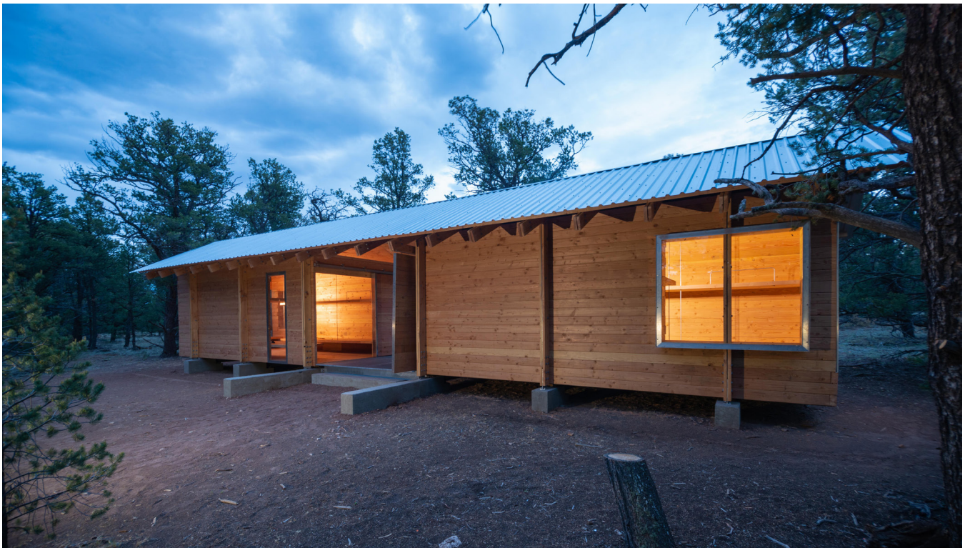
Figure 1. Exterior image of one of the six Cottonwood Gulch Cabins designed and built by ColoradoBuildingWorkshop. Image credit Jesse Kuroiwa.
