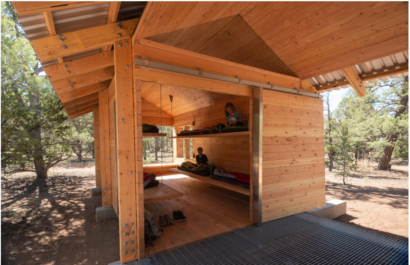
Figure 3. Interior of the Cottonwood Cabins. The SLT is visible in the wall, floor, ceiling, doors, and bunk beds of the cabin. Image credit Jesse Kuroiwa.
