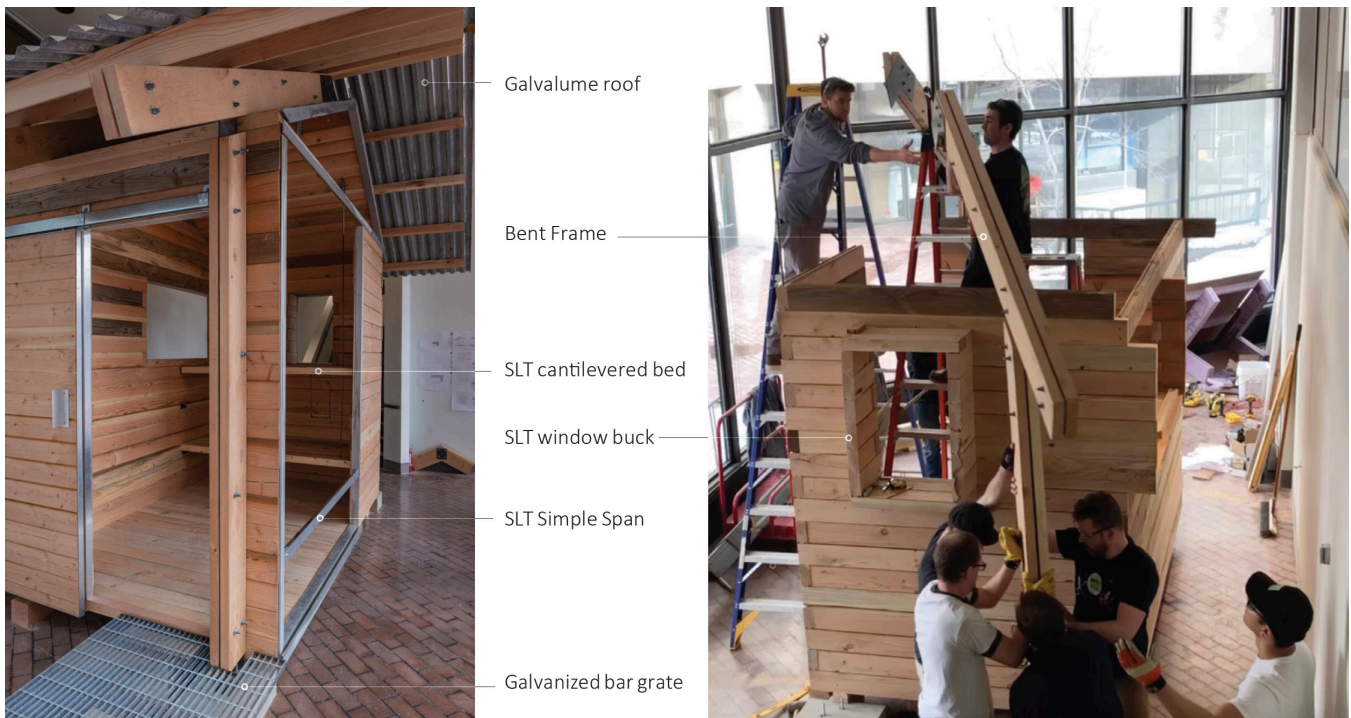
Figure 10. Two views of the 1:1 proof of concept mock-up built prior to the start of the cabin construction. The students used the design exercise to gather critical information about tolerance, materials, detailing, and construction sequencing. Image credit Rick Sommerfeld
